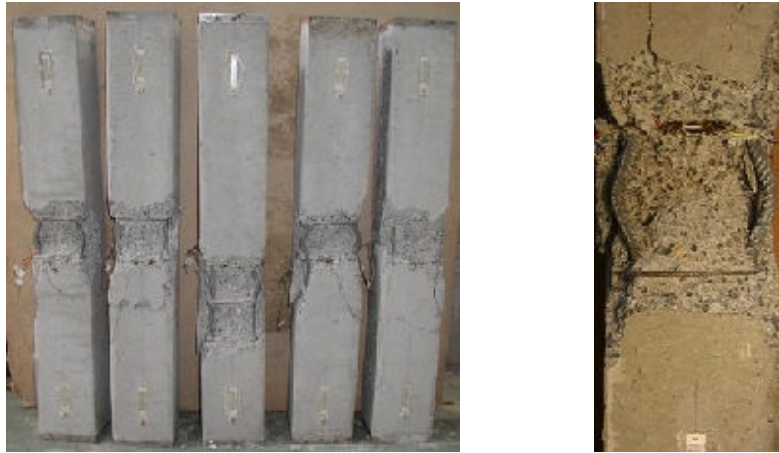
Fig. 2 Experiments: Series N10 after collapse (left). Front view on the damaged zone at the midheight of the column (right).
