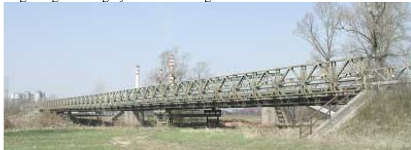
Fig.1 General view on the bridge
