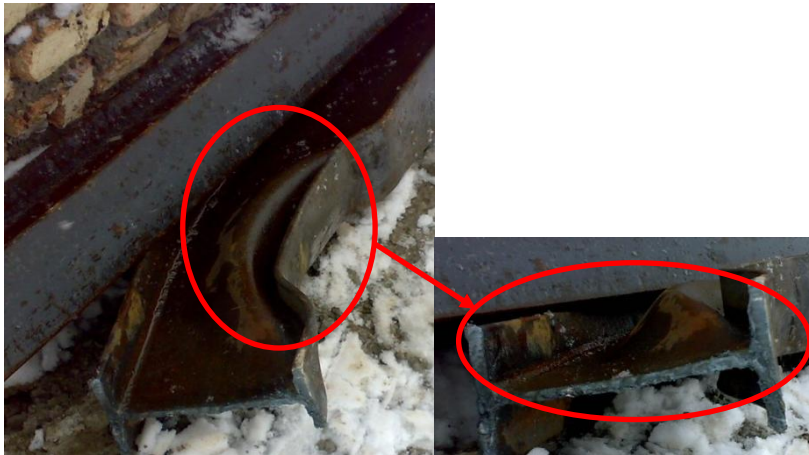
Fig. 8. Buckling of beam web during bending
