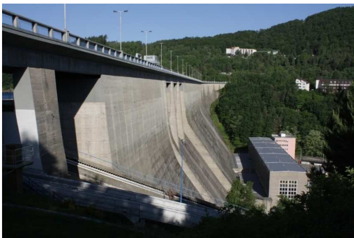
Fig. 1. Gravity concrete Orlik dam
