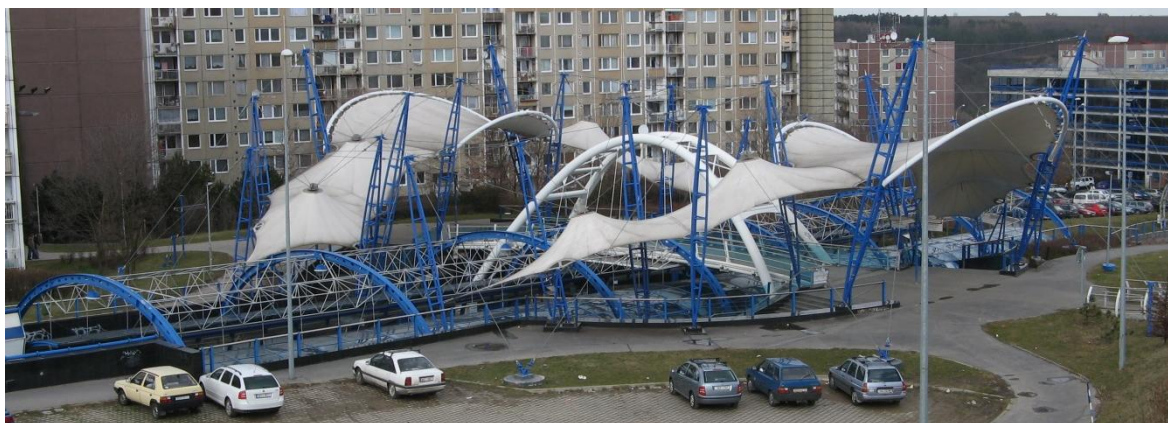
Fig. 1 The overview of the tension fabric roof of the tram stop “K Barrandovu” in Prague.
