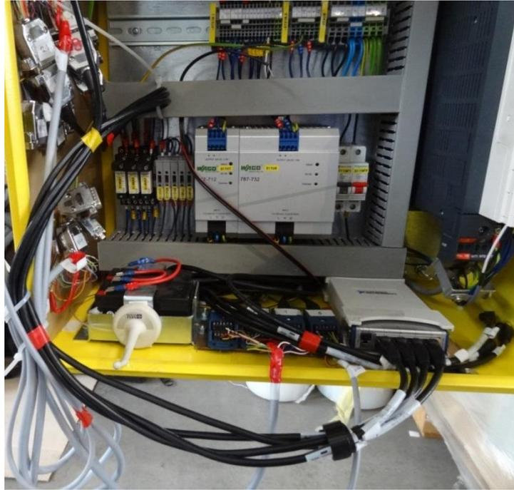
Fig. 6: Chassis cDAQ in switchboard of rotation ring.
