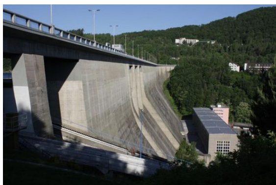
Fig. 3: Gravity dam's body of the dam Orlik.
