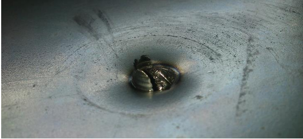
Fig. 3: Failure mode of a broken sleeve. Specimen shown from below.
