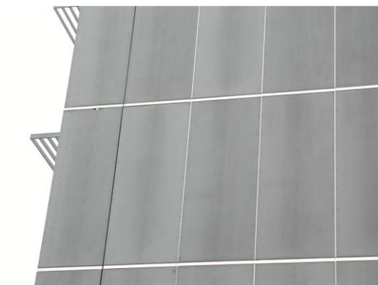
**Fig. 2** Cembonit FDA cladding sheets
