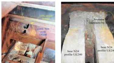
**Fig. 1** Typical examples of corrosion damages in supporting structure of steam boiler
