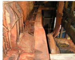
**Fig. 2** Lost of stability connected with plastic deformation
