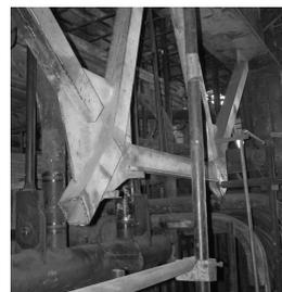
**Fig. 5.** Removed struts from left side of boiler (U-profile web is on right side).
