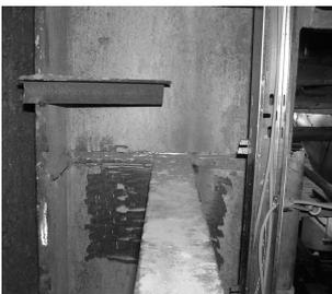
**Fig. 4.** Joining of U-profile to the column S2L.
