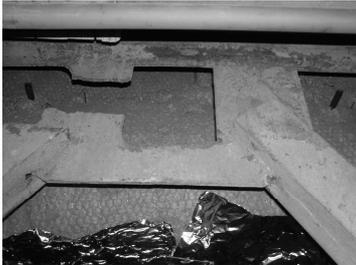
**Fig. 2.** Burned-out of framework joint sheet.
