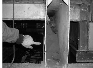
**Fig. 3.** Deformed webs of beam.
