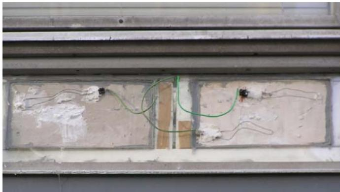
**Fig. 4.** Gypsum blocks in the building envelope, the view from the outside
