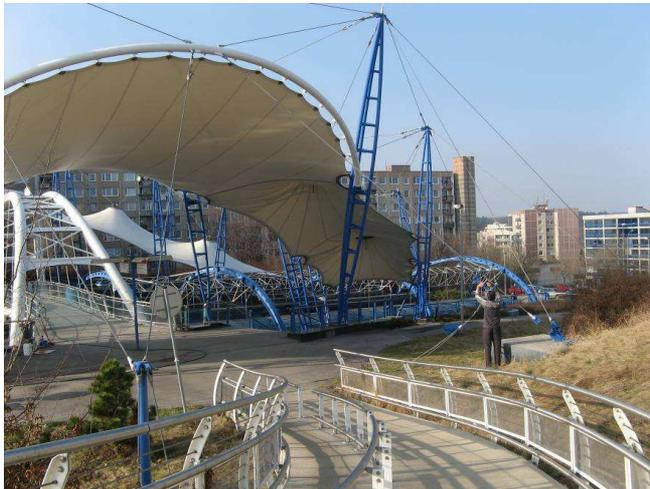
**Fig. 2.2** The application of equipment for the cable forces measurement
