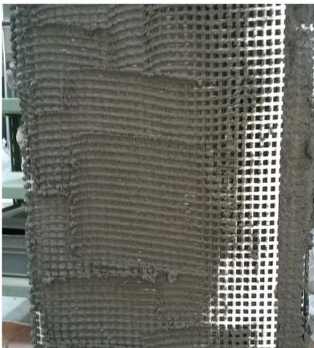
Fig. 3: Application of TRC on brick masonry column's surface.
